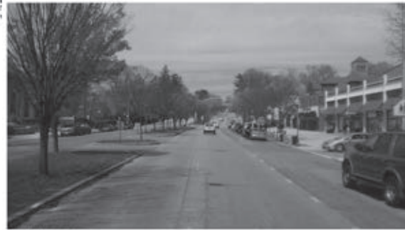
EXISTING CONDITIONS Roland Avenue and Colorado Avenue Intersection Looking North
