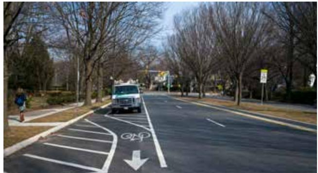
Bike lanes shift adjacent to vehicle lanes at bus stops. This movement can be surprising to passing motorists.
