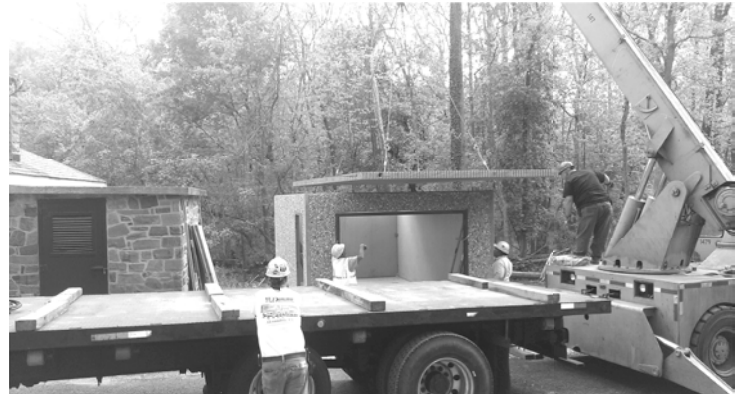
Workmen prepare to lower the roof onto a new storage shed near the ranger station in Robert E Lee Park. Photo: Siobhan O'Brien Budnitz
