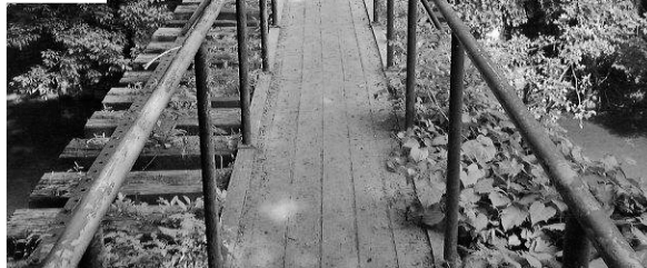
The planking on the trestle over the Jones Falls, which shows gaping holes, will be replaced with wider decking. Handrails will also be added.
