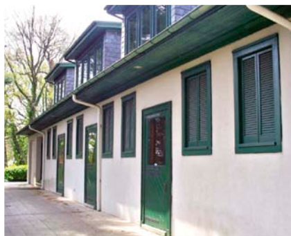
During the meticulous renovation, the exterior stall doors were duplicated and replaced.
