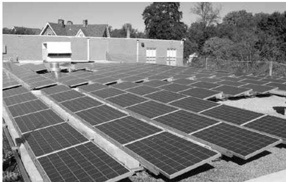
RPCS installed a 35.88-kilowatt photovoltaic solar array on the roof of the Jean Waller Brune Lower School. Photo courtesy of RPCS
