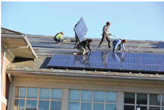
The work crew retrofitted a classic slate roof for the installation of a large solar array. Photo courtesy of Gilman School
