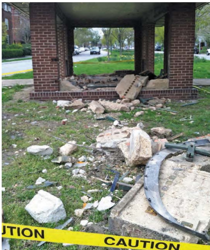
The 2013 collision caused severe structural damage. Photo courtesy of Stacy Montgomery, CHAP.
