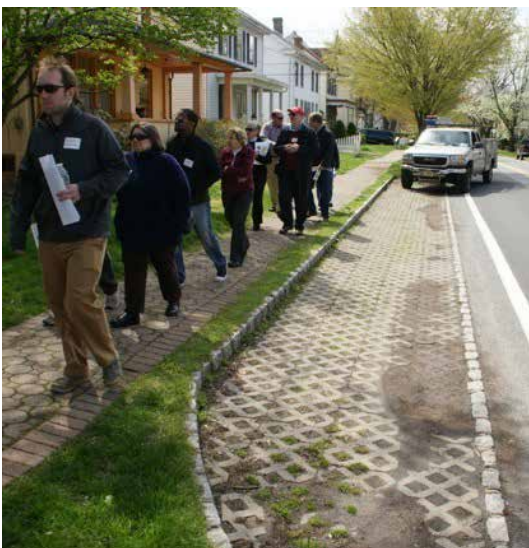
Example of parallel parking on permeable pavers
