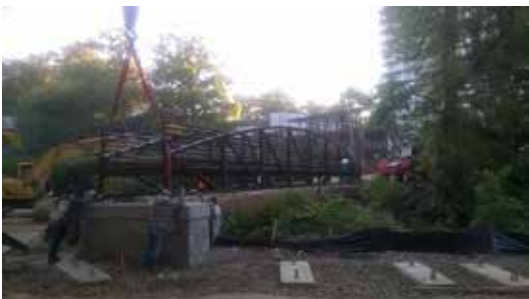
Pedestrian bridge construction
