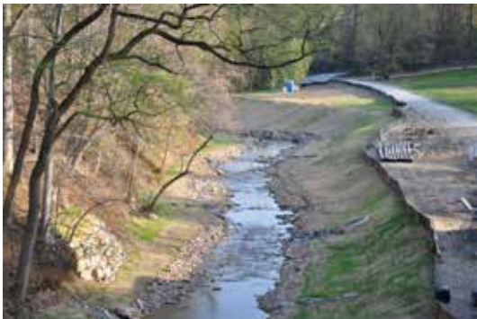
Lower Stony Run stream restoration project
