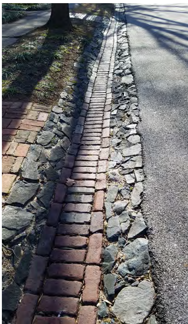
Pervious gutters allow stormwater to seep into the soil. Photo: Devra Kitterman
